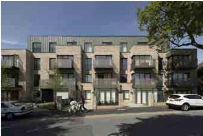
Upper Floor Recess & Definition
