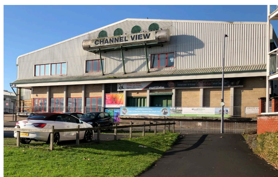
Channel View Leisure Centre | Canolfan Hamdden
