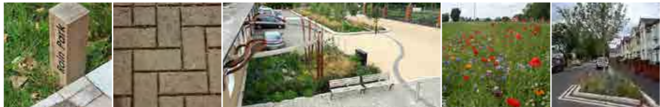
Rain park signage Limited Permeable Paving where there is no 'green' alternative SuDS linked through hard landscape and Living Streets Annual meadow transition space into The Marl and SuDS basins Rain garden build outs within Living Streets and traffic calming
