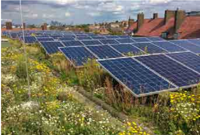
Green Roof Solar
